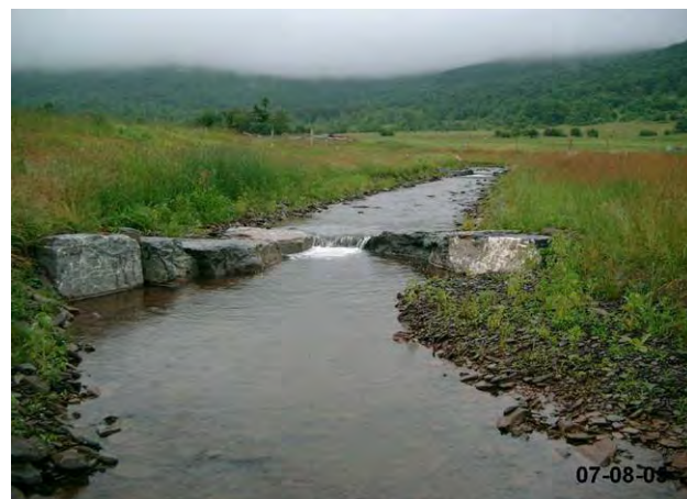
Figure 3.17 Rock Cross-Vane
