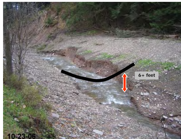
Figure 3.20 shows downcutting after dredging.
