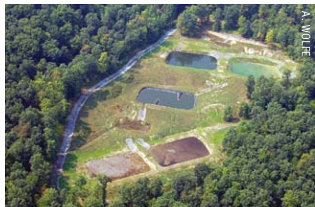
Middle Branch passive treatment system
